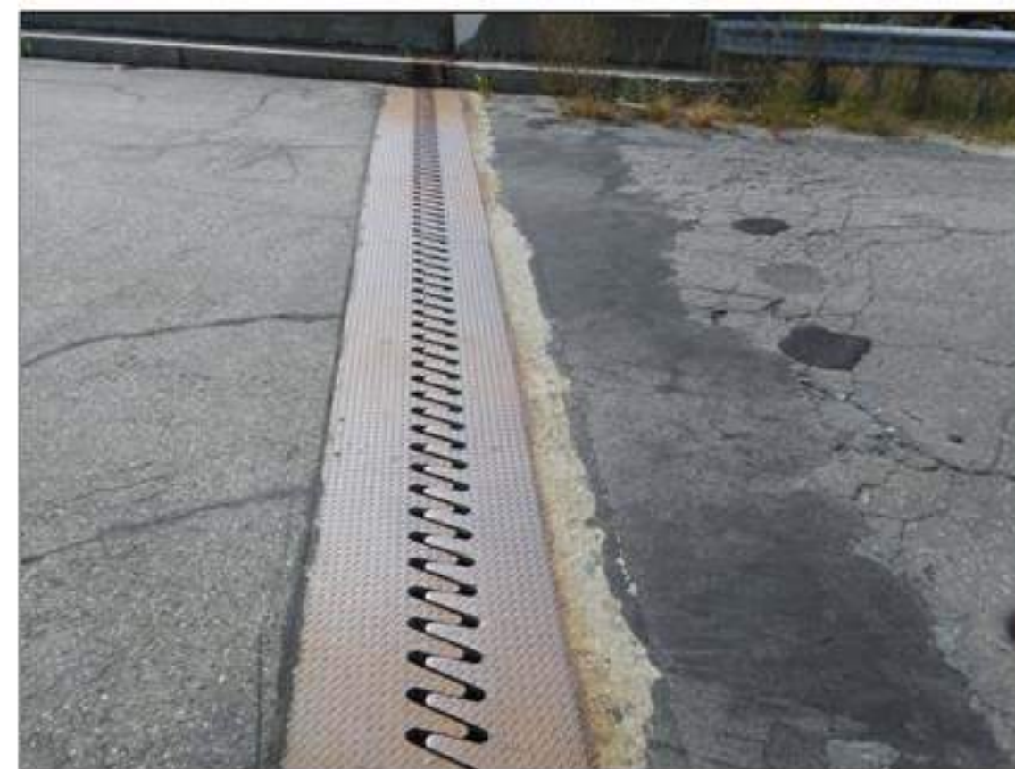
West finger joint with patched approach pavement
