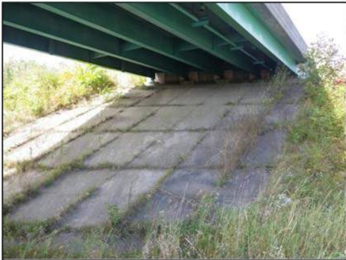
West abutment slope protection
