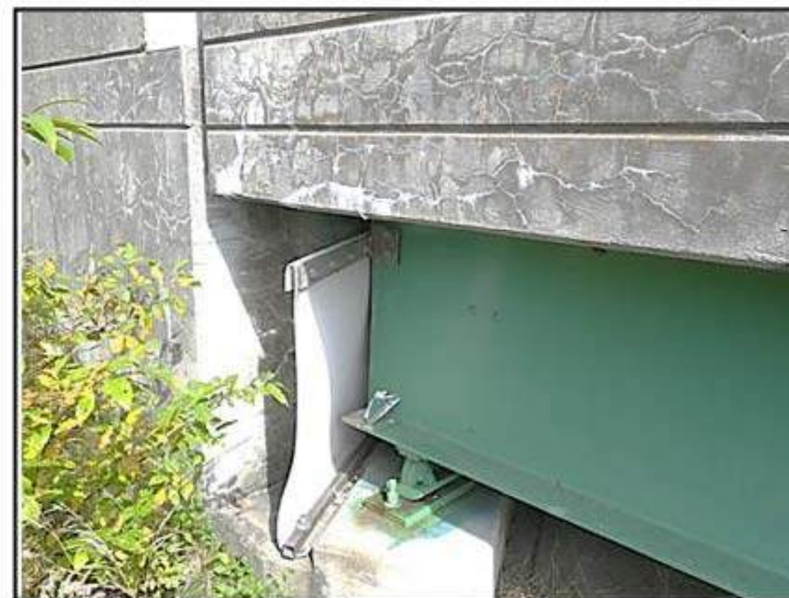
Cracking and efflo at the SW corner
