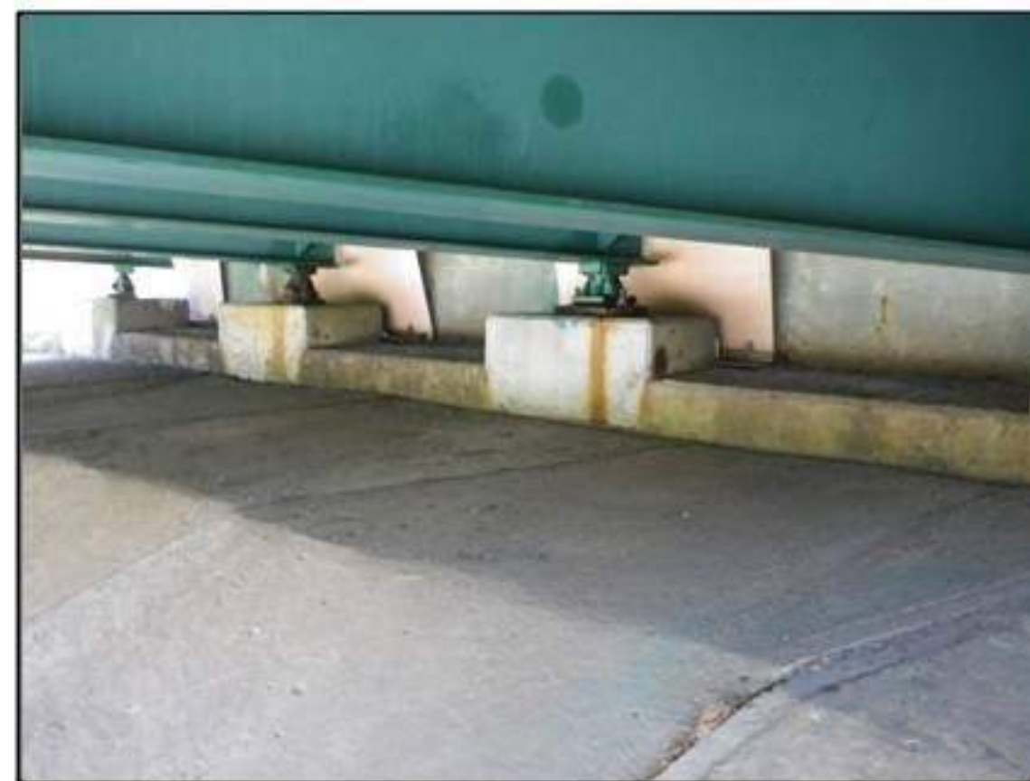
East abutment bearing and "mud flap" protection
