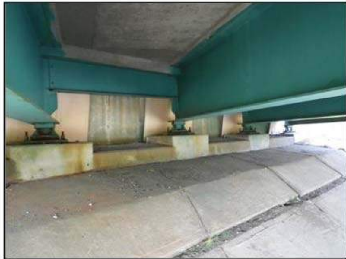
West abutment bearings with "mud flap" protection
