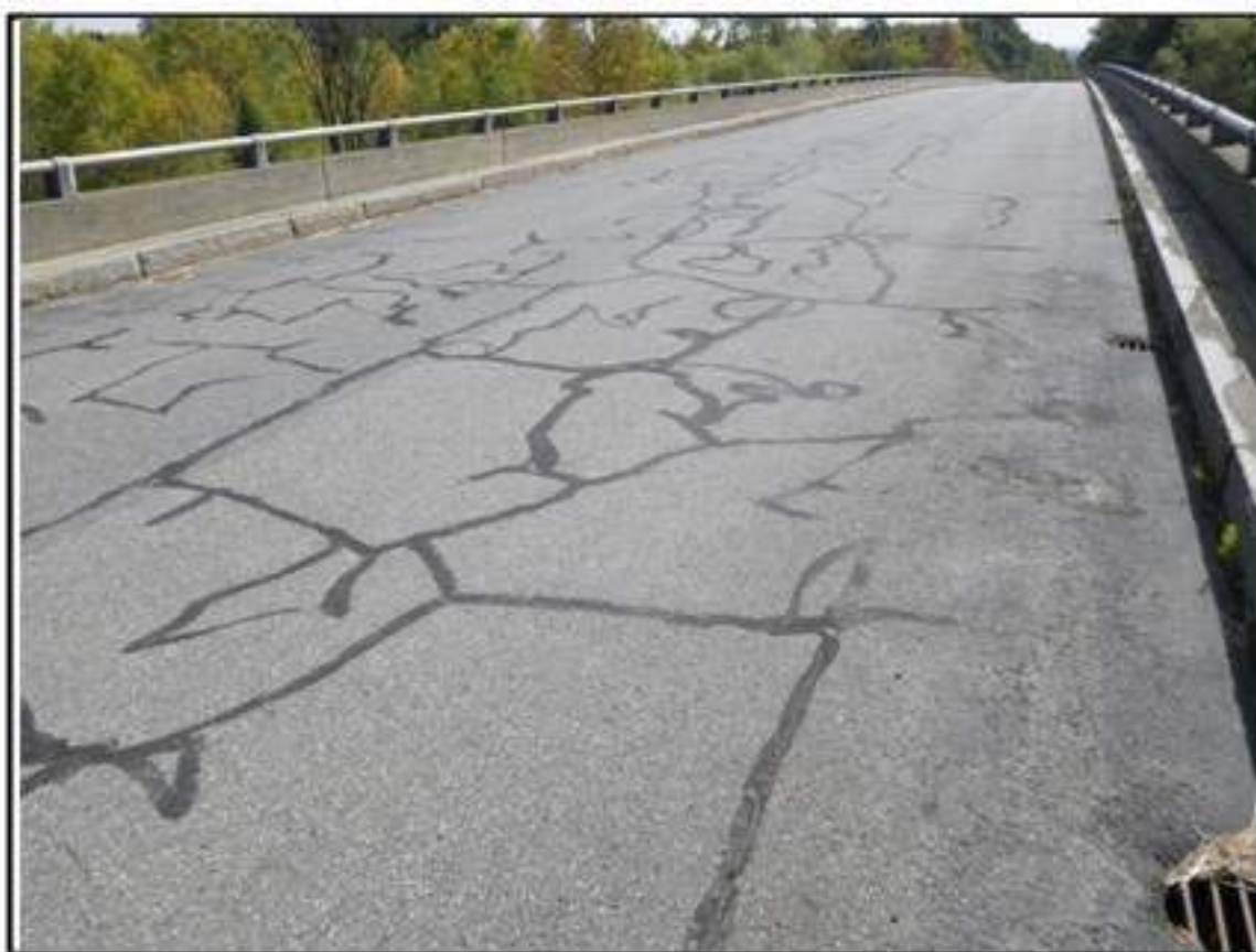
Cracked and sealed bituminous wearing surface
