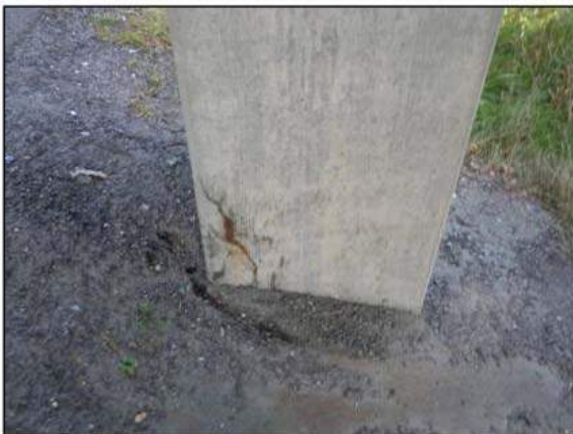
Isolated areas of concrete column cracking and rust staining
