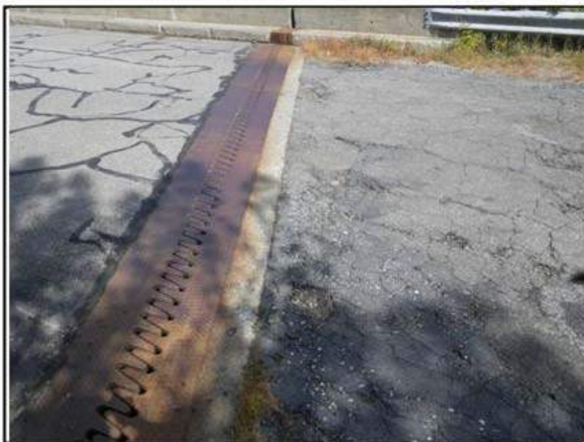
East finger joint and approach pavement in poor condition
